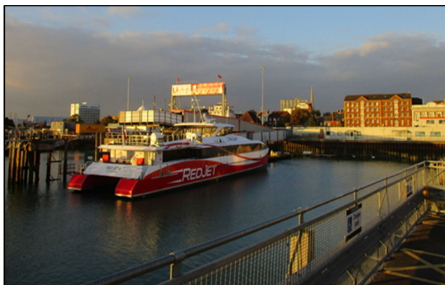
Fig. 2 Port and coastal infrastructure at Southampton
